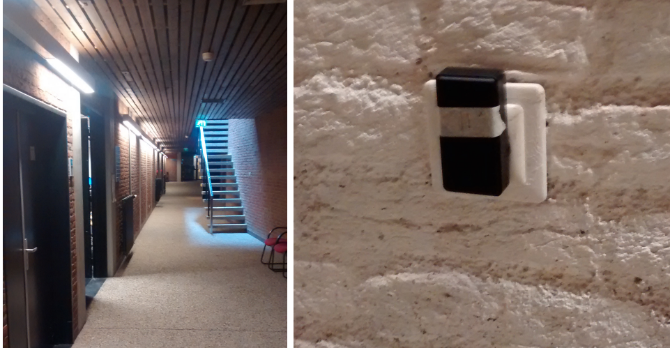
Figure 4.3.3: The basement of the Faculty of Social Sciences at the Radboud University was used as a test for larger environments. In total, fourteen landmarks were placed in wall sockets (right picture).
